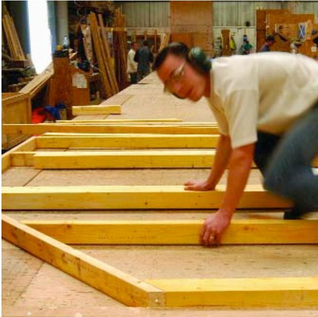
Constructing a timber frame in a factory
