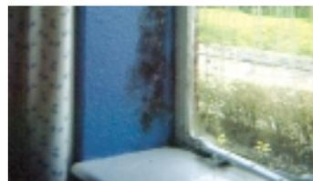
A local drop in the surface temperature around openings, or 'Thermal Bridging', can give rise to unsightly mould growth and damage to reveal finishes.
